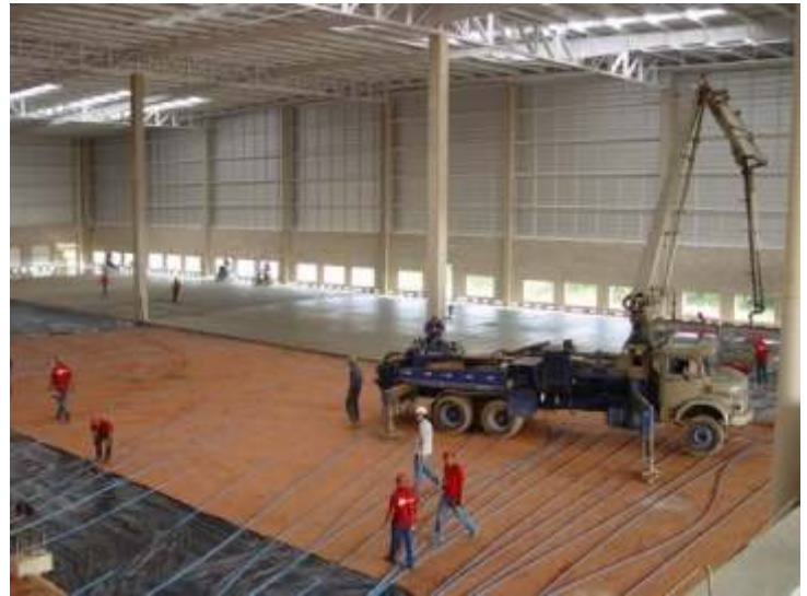
Facility under Construction
